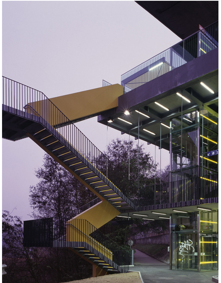
Neubau RBS Station Felsenau Bern Ebene Felsenau-Viadukt
