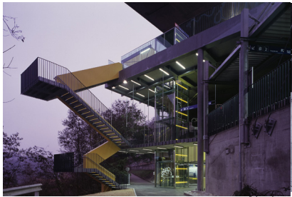
Neubau RBS Station Felsenau Bern
